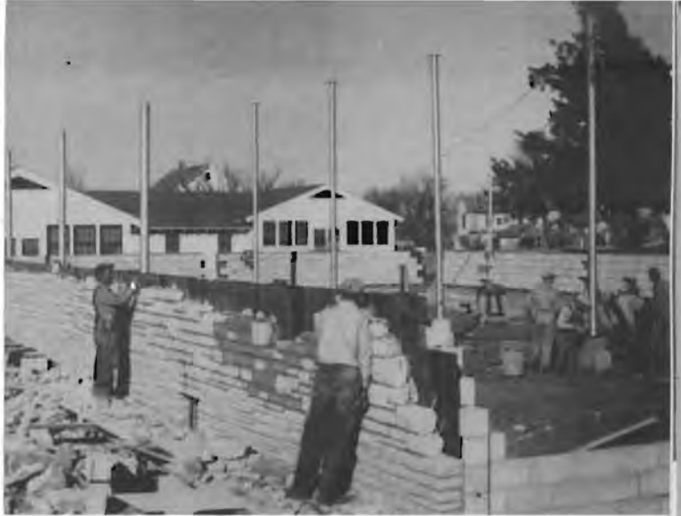
The steel's up. It won't be long now.
