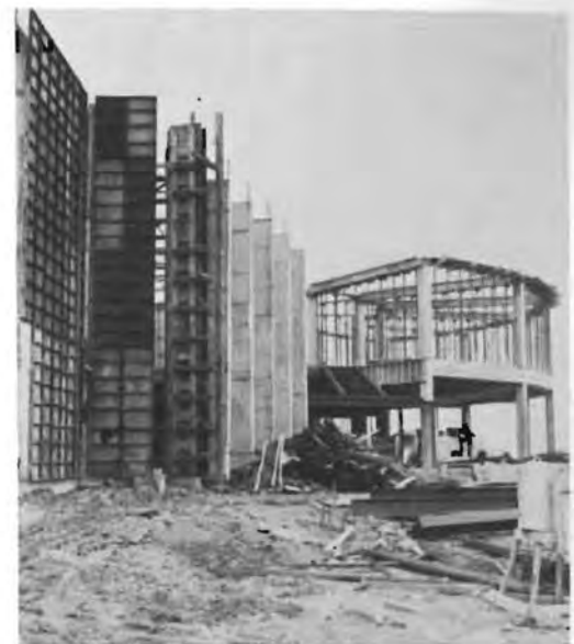
Walls go up for the recital hall.
