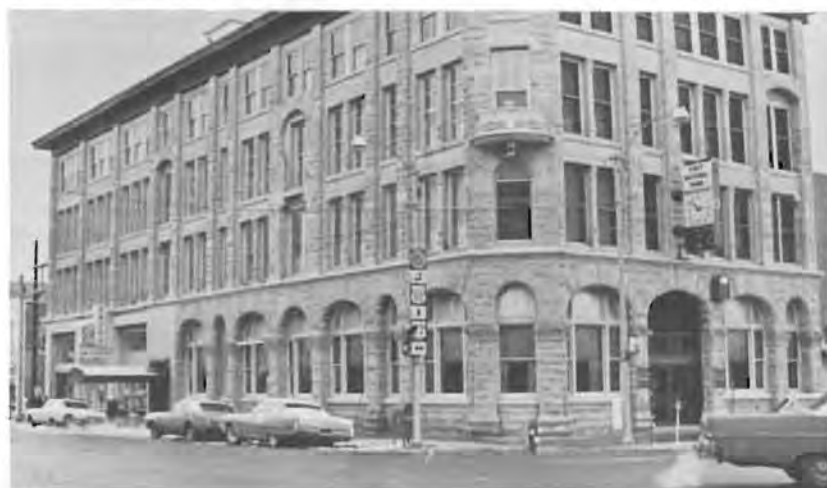
The Time and Temperature Corner
